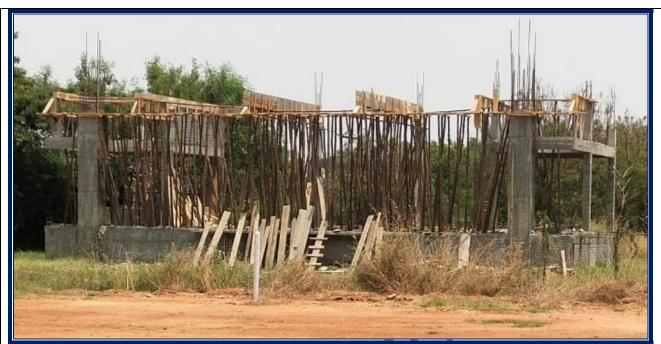
**GS-ANC Open Air Auditorium Construction under progress** Base of the Stage Height – 6 feet- Centering work getting completed. Ready for Ceiling Roof Concrete – Status as on 31-03-2021
