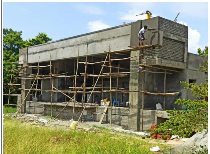
**GS-ANC Open Air Auditorium** – Construction is completed. Flooring, Plastering, plumbing, painting, electrical fittings are yet to be carried out. Planning to inaugurate in a couple of months.
